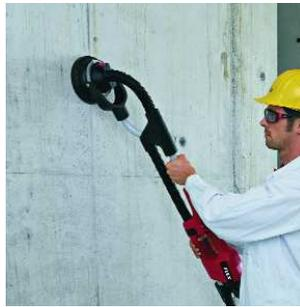
Concrete joints or concrete ridges are easily reached and quickly eliminated
