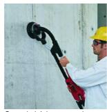
Concrete joints or concrete ridges are easily reached and quickly eliminated
