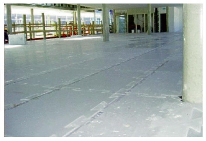
Patented cover sheet with clip-system helps for quick and easy installation!
