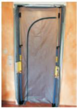
This dustproof door can be guickly and easily assembled using two scaffolding poles.
