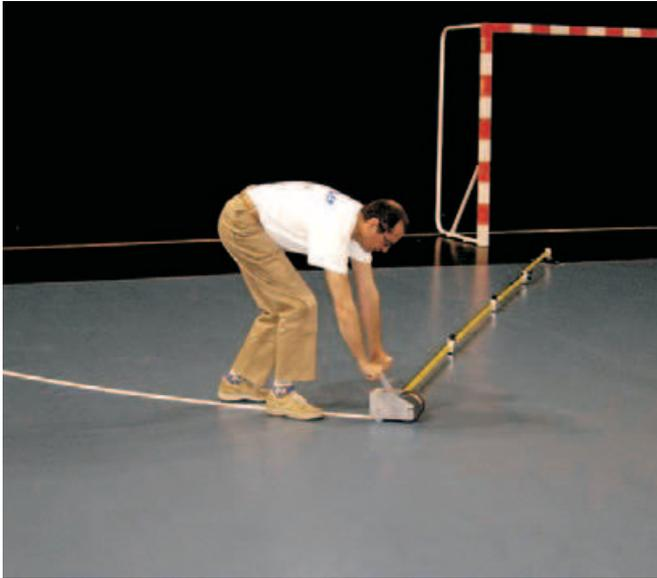
Two parallel tapes can also be applied with the device.
