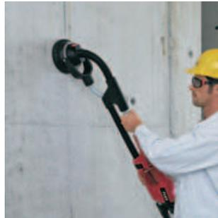
Concrete joints or concrete ridges are easily reached and quickly eliminated even in rooms with high ceilings.
