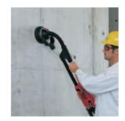
Concrete joints or concrete ridges are easily reached and quickly eliminated even in rooms with high ceilings.
